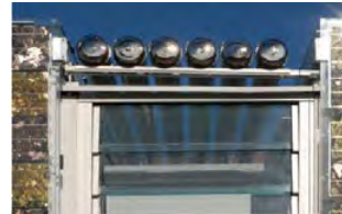
Figure3. PVT collector and vacuum collector of HFT
