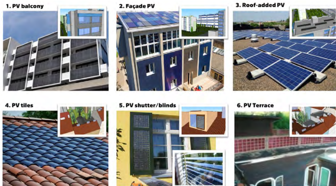
Figure 2. Examples of architecturally integrated PV systems in the two building blocks: (1) PV balconies. Source: Etsprojects; (2) Coloured PV-façade. Source: Swissinsio; (3) Roof-added PVs. Source: Cromwellsolar; (4) PV tiles. Source: Tradeford; (5) PV shutter and PV blinds. Source: COLT international, Solargaps; (6) PV terrace. Source: (López and Frontini, 2014).
